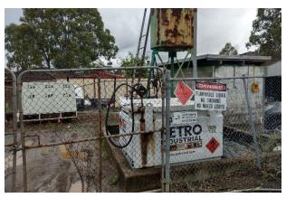
**Photograph 16:** Petrol and diesel ASTs within dedicated concrete bunded area.
